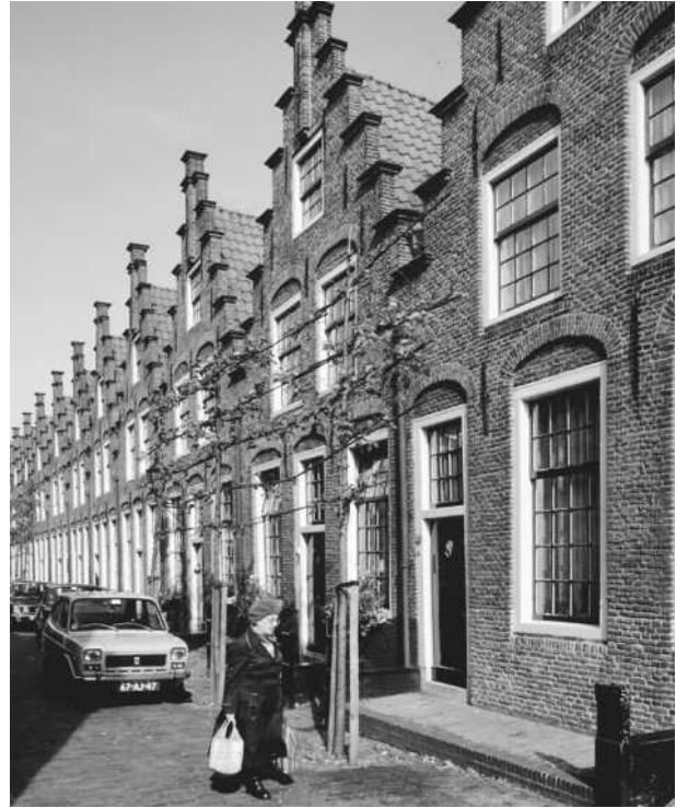
Brick row houses in Haarlem have prominent front doors and large windows.
